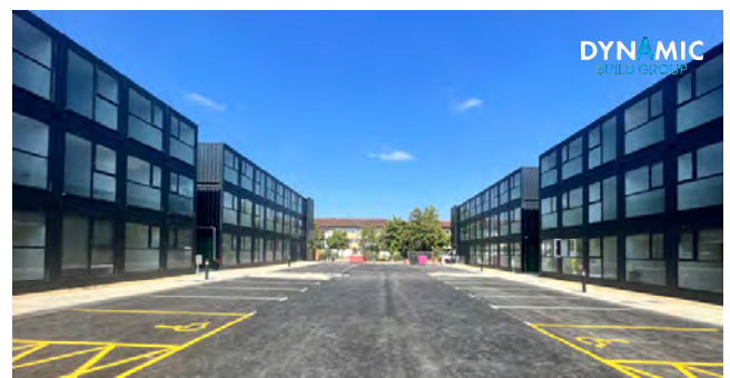
Dynamic Build Group - Modular housing project at completion
