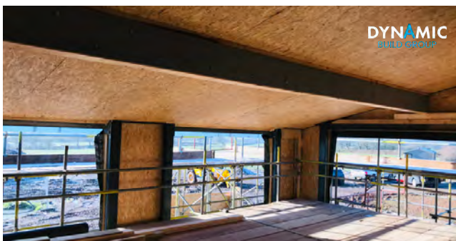
Dynamic Build Group - SIPs custom build during installation
