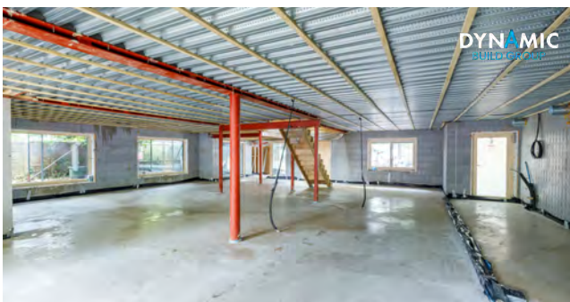
Dynamic Build Group - ICF self build project during installation
