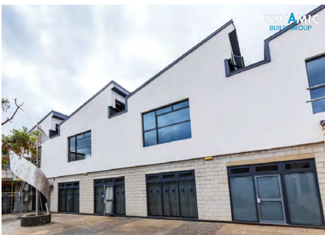
Dynamic Build Group - Education project
