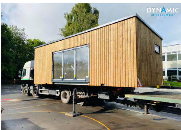
Dynamic Build Group - Volumetric Modular education sector project
