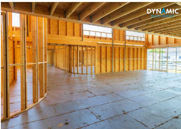
Dynamic Build Group - Timber Frame with panelised floor and roof system
